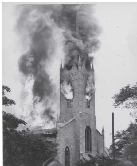
A fire devastated Chillicothe St. Peter Church on June 20, 1947, causing $250,000 in damage. The side walls were saved and incorporated into the rebuilt church. Photos courtesy St. Peter Church
