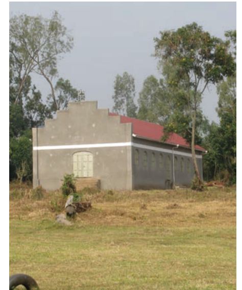
Exterior of the chapel at the Miryante orphanage.
