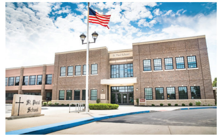
Westerville St. Paul School has added a second floor which expands the building by 26,000 square feet. Photo courtesy St. Paul School
