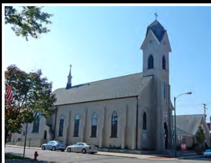
Front Page photo: London St. Patrick Church is celebrating the 150th anniversary of the church building and the parish itself. The parish center (right) was built in 1999.
