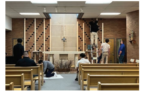
Students work on the chapel transformation.
