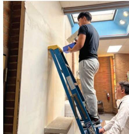
Drywalling was one of the skills the students learned.
