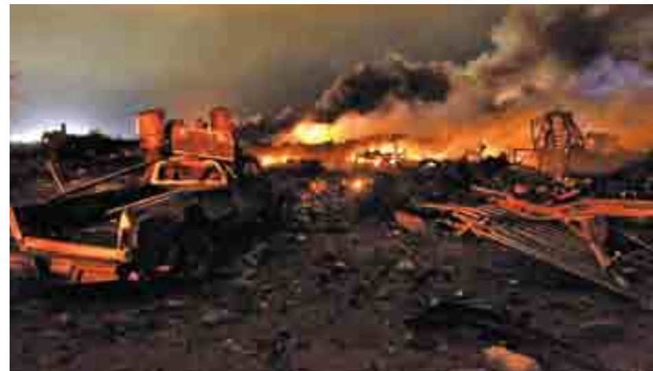
A vehicle is seen near the burning remains of a fertilizer plant in West, Texas, on April 18 after an explosion there the previous day. Rescue workers searched rubble for survivors of the explosion in the small town near Waco that killed as many as 15 people and injured more than 160 others. CNS photo/Mike Stone, Reuters
