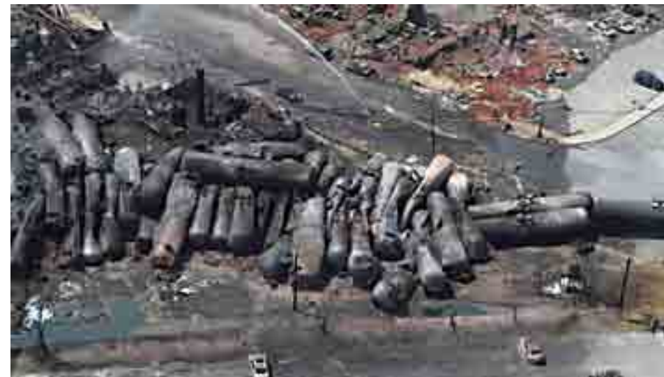
Burned train cars are seen in this July 8 aerial view following a derailment and explosion in Lac-Mégantic, Quebec. Most of the town's central business district and dozens of residences were destroyed on July 6 after a runaway train that was headed to a New Brunswick oil refinery derailed and exploded. CNS photo/Transportation Safety Board of Canada via Reuters
