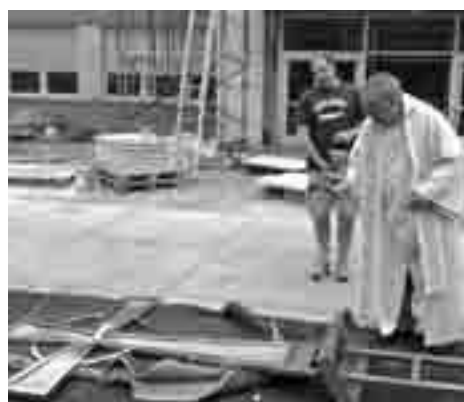
CROSS BLESSING Father Raymond Larussa of Columbus St. Matthias Church blesses the new cross that sits atop the renovated front entrance of Columbus St. Francis DeSales High School. The cross was modeled after the pectoral cross of the school's patron saint. Scott Hartman, the school's director of advancement and business operations, is in the background. Several other faculty and staff members witnessed the blessing two days before school started and signed their names to the structural support of the cross. Photo courtesy St. Francis DeSales High School
