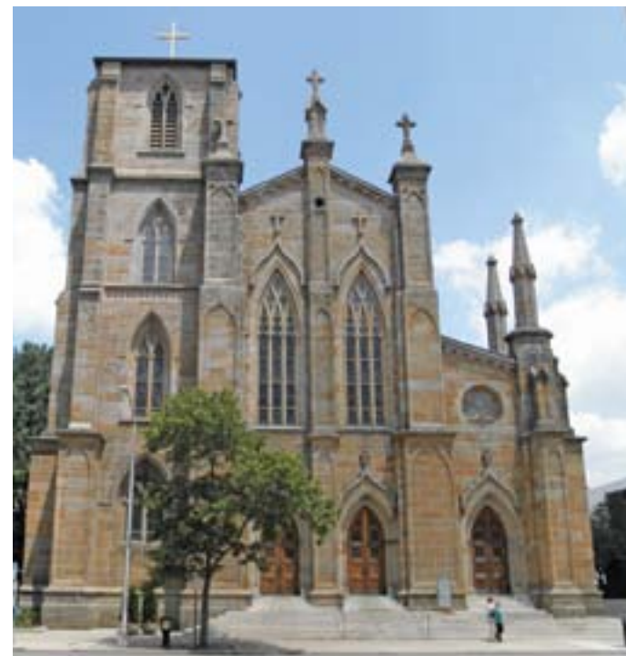
Above: Exterior view
