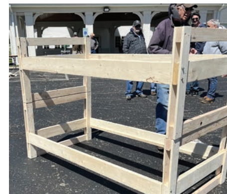
A bunk bed under construction
