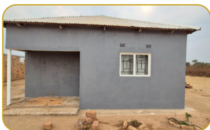
A 6.2 kV solar system brings light to the home
