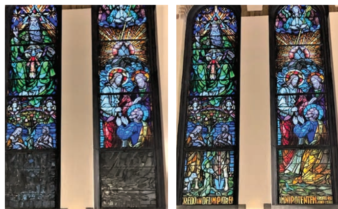
Stained glass windows at Columbus St. Aloysius Church are shown before and after recent restoration work.
