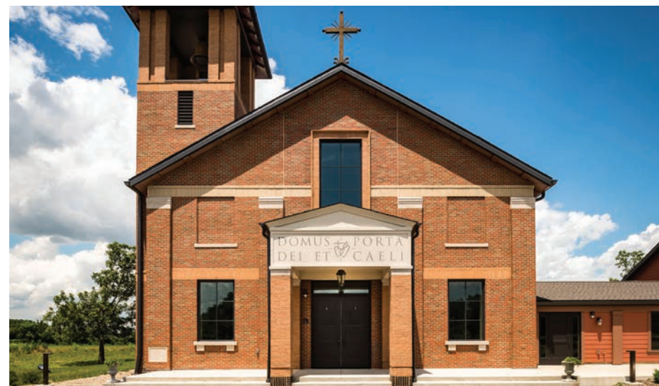
Cardington Sacred Hearts Church, designed by Columbus architect William Heyer and dedicated in 2015 to replace a church that burned down in 2013.
