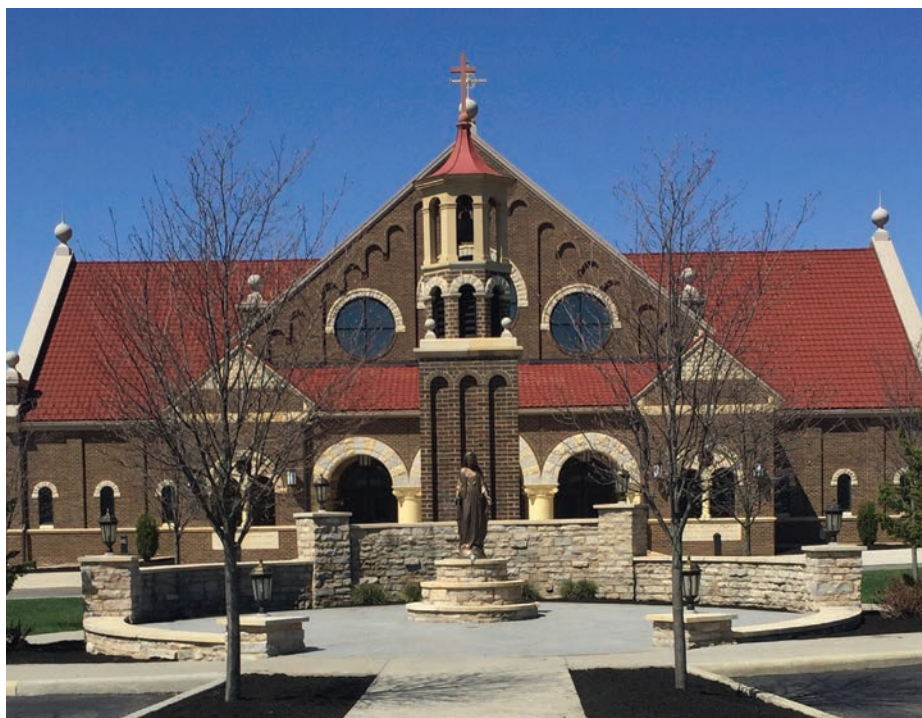
Westerville St. Paul Church, dedicated in 2011 and designed by David Meleca, is the largest church in the Diocese of Columbus. The 37,000-square-foot building's sanctuary can hold about 1,400 people.
