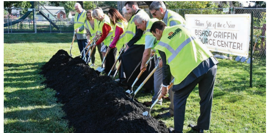
Participating in the groundbreaking for the Bishop Griffin Resource Center are (from left) Jim Cetavich (Ruscilli Construction), Casey Byrnes (Triad Architects), Tammy Tucker (Mid Ohio Food Collective), JoEllen Gohr (board member), Nancy Roberts-Moore (executive director), Bishop Griffin, Father David Schalk, Pat Kelley (Co-Chair, Lift Up Your Neighbors Campaign) John Igel (CEO, Igel Construction) and Tony Ruscilli (CEO, Ruscilli Construction).
